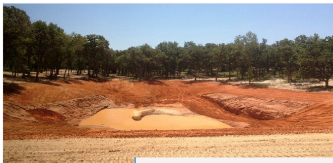
Figure 3. A pond during construction.
